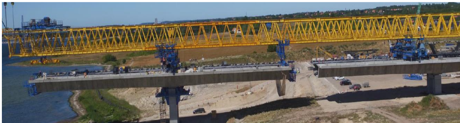
BALANCED CANTILEVER: FROM SEGMENT "04D-U" TO "13D-U"
