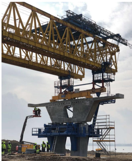
Erection of pier segments S00D and S00U on temporary jacks.
