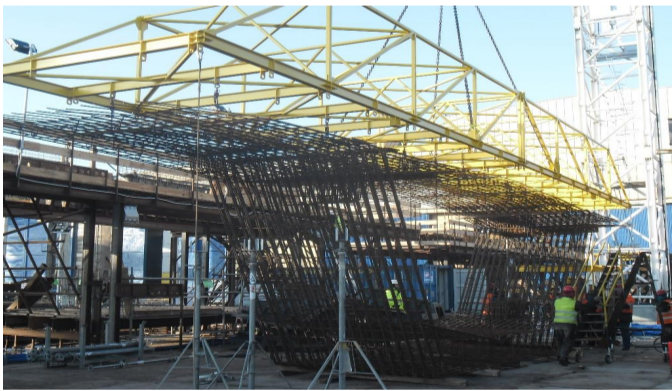
REBAR CAGES ASSEMBLY
