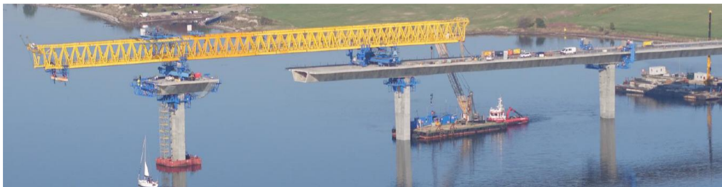
BALANCED CANTILEVER: UNTIL PAIR OF SEGMENT "03.D – 03.U"
