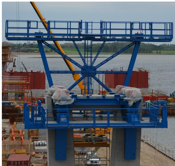
Installation of pier brackets before segments erection.
