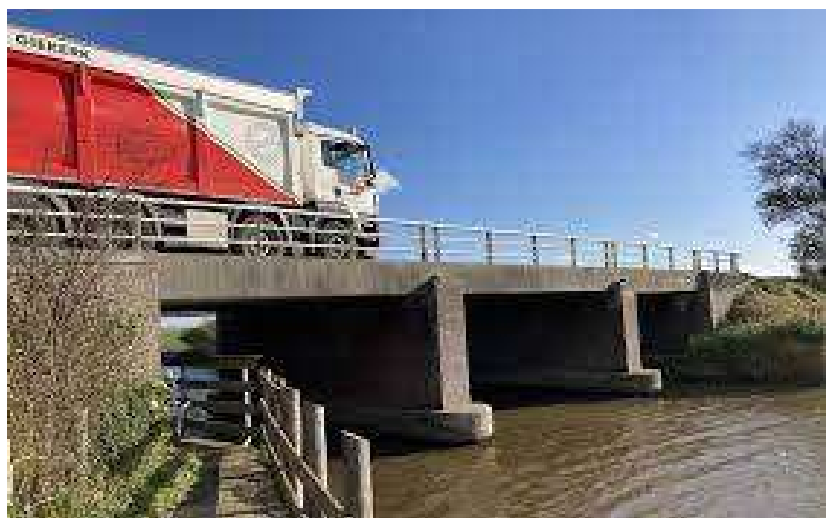
Kowebrêge, N358 Road in Friesland Province
