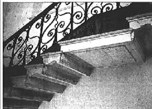
Fig 16. (Below left) Diagram showing the deflected shape of a rebated flight (courtesy Ian Russell). Fig 17. (Below) Landing within a flight of the Beauty Stair at Hampton Court (photo courtesy Sam Peles).
